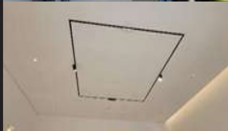
Construction at Al-Ansab Heights in Bousher
